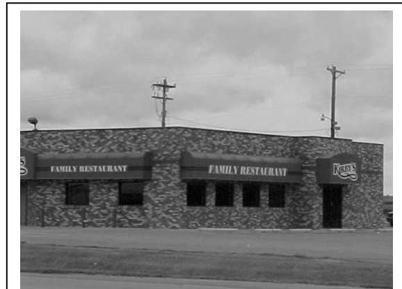
Sign, Architectural Canopy Sign, Awning or Canopy
